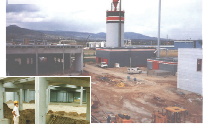
1988 - The construction of U1
